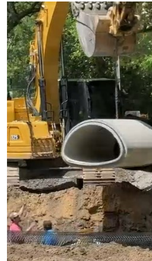
Improvements being made in Pascagoula.
