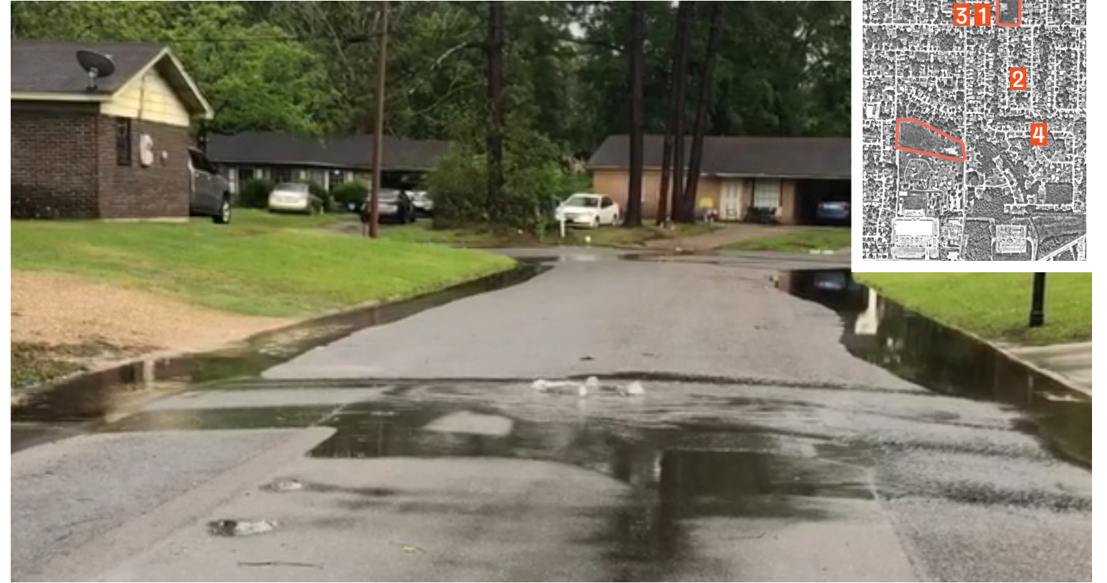
2 | Overflowing storm sewer on Rose Drive (and Winona Drive)
