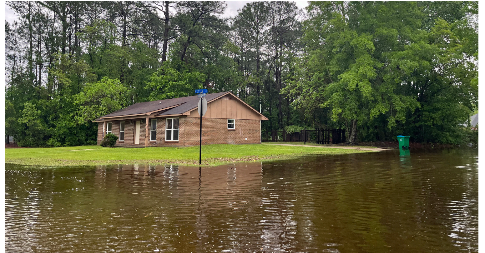
4 | Intersection of Vester Lane and Morningview Drive
